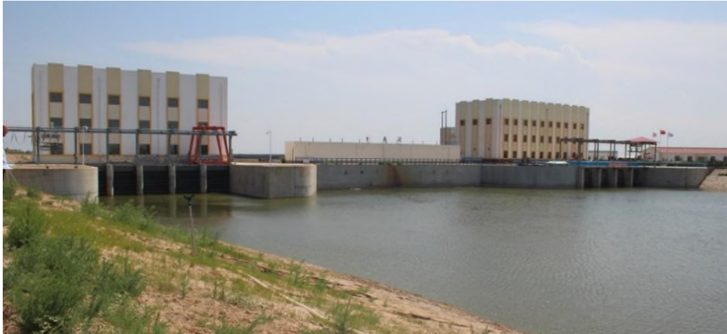
Figure 3. Discharge sluice and drainage pumping station of Hetao Irrigation District and Ulansuhai Lake to Yellow River
