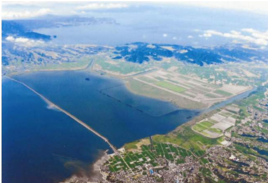
Figure 5. Aerial view of Isahaya Polder and its surroundings (Ota, 2016)
