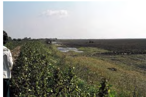
Seepage spots at the inner too of the dike surrounding the Pardina Polder in the Danube Delta
