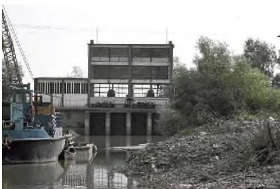
Pumping station of the Pardina Polder in the Danube Delta. This pumping station can be operated on supply and on discharge
