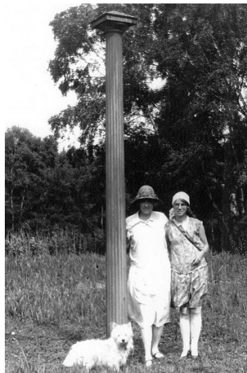
Figure 3. Holme Post installed in 1851 at surface level when Whittlesey Mere was drained (source: County Record Office, Huntingdon)
