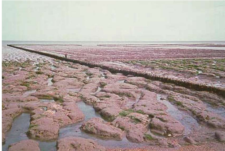
Figure 7. Brushwood groyne perimeter fence enclosure to enhance natural sedimentation in the Dengie Flat, south-east Essex (Source: Colenutt, 1999, picture D. Carter).
