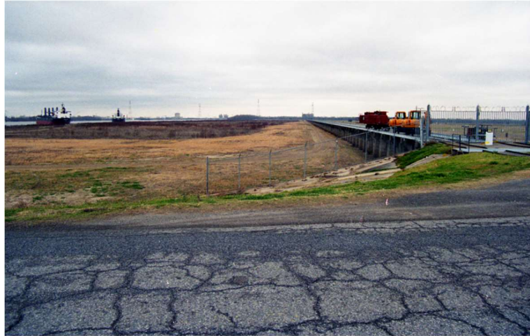
Figure 4. The Bonnet Carré Spillway 19 km upstream of New Orleans to divert flood water from Mississippi River to Lake Pontchartrain
